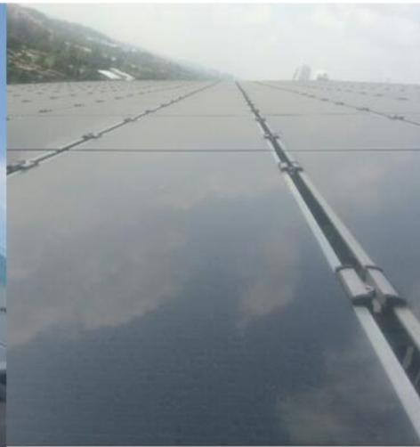
*Figure 6 & Figure 7 Thin-film photovoltaic solar cells*
